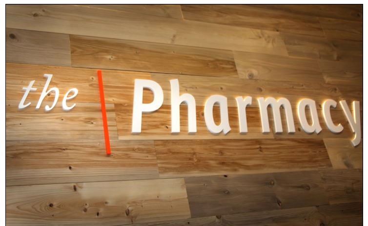
The natural wood used in the Pharmacy design, seen here, was culled from the Penobscot River. Old logs that had settled at the bottom of the river, back when the waterway was used for shipping, have been “reclaimed” and used in construction.
