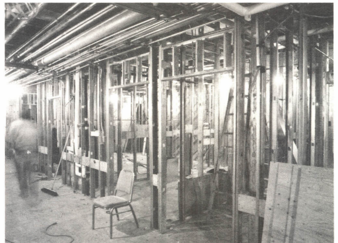
BY FEBRUARY , the walls were studded, as seen in the corridor, above, and fireproofing was prepared and applied to columns and beams, below.
