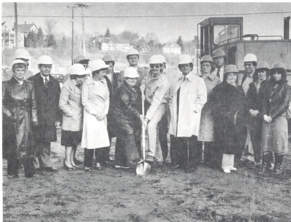
GROUND BREAKING CEREMONIES for the new home of the Medical Services Federal Credit Union were held November 30. The building will be located at the intersection of Park Avenue and Forest Street, about two blocks from the hospital. Above, MSFCU Board Chairman George A. Drew and Building Committee Chairman Jeannette Fournier break ground. The building is expected to be finished early next summer. (A/V Photo)
