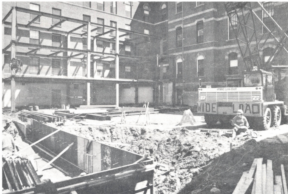
THE STEEL FRAMEWORK for the three-story section of the Bypass Corridor is in place in the Food Services courtyard. When completed the "bypass" corridor will be the main corridor of the hospital on the ground floor.
