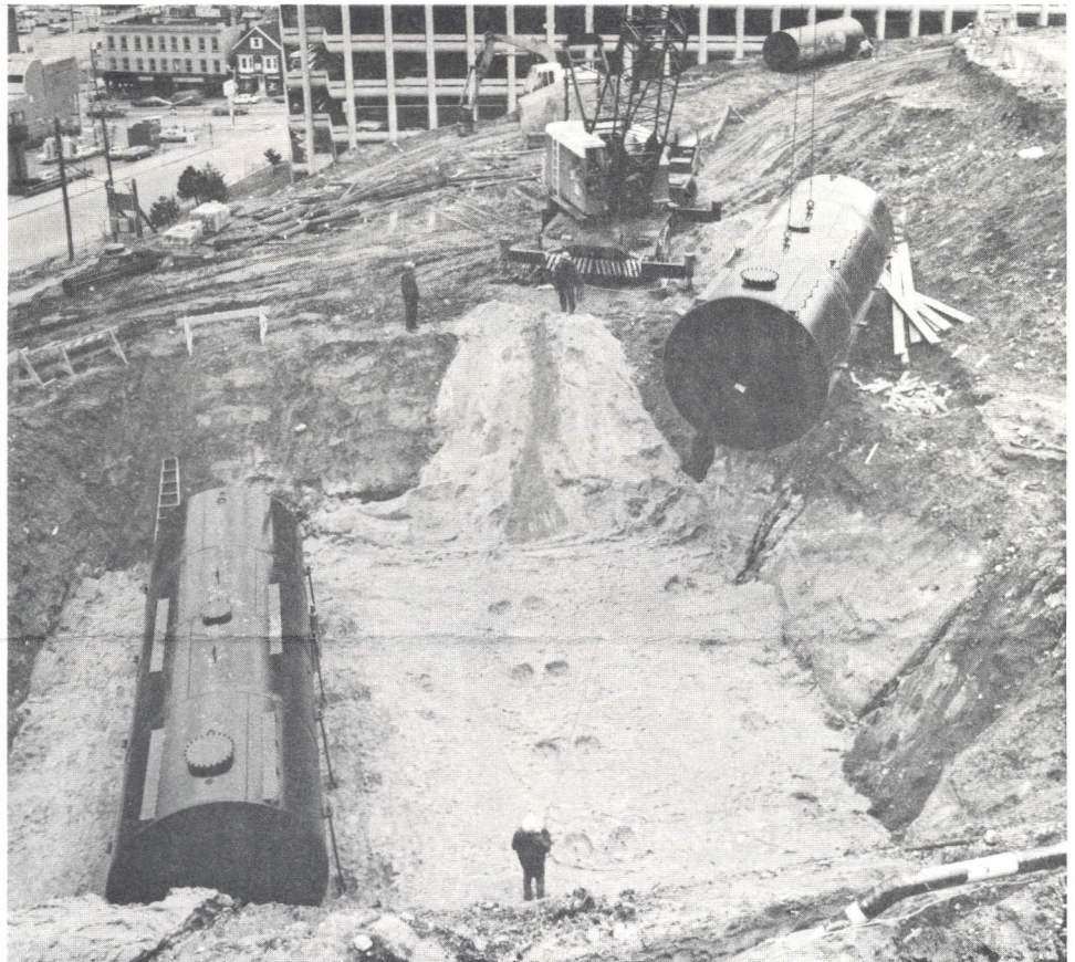
THREE 20,000 GALLON OIL TANKS were swung into place behind the Engineering Services Building last week. They will hold #4 fuel oil for the hospital's boilers. Above left, workers close the mid-point gap in the sheltered walkway leading to the parking ramp. All traffic to the construction site will now use the lower road. (A/V Photos)
